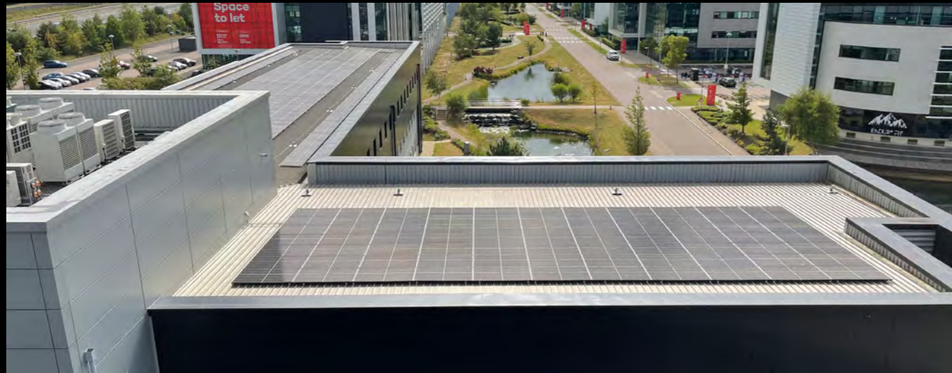
SOLAR PANEL INSTALLATION AT DAKOTA EUROCENTRAL
